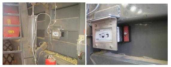
The picture below shows the inside of the channel. The metal strip welded to the wall before the TX/RX unit minimizes buildup of material around the TX/RX units that might damage them.
